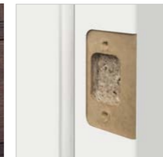
STRIKE PLATE preparation for standard 2 1/4" strike plate
