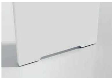
PASS-THROUGH VENTILATION UNDERCUT *) undercut 15 mm - for rooms with recuperation undercut 26 mm WC for doors 80'-100' *) undercut 38 mm WC for doors 60'-70' *)
